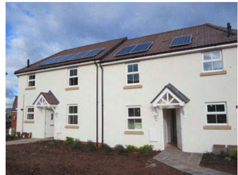
Picture 12 Photo-voltaic roof panels
