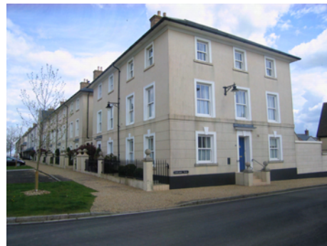
Picture 28 Taller, continuous frontages along the main street
